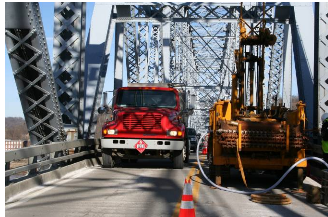
The bridge has two 10 foot lanes
