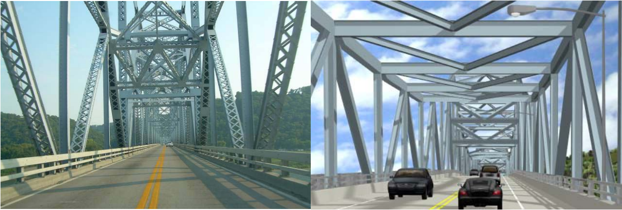
Figure D.7 – View along Highway crossing Bridge
