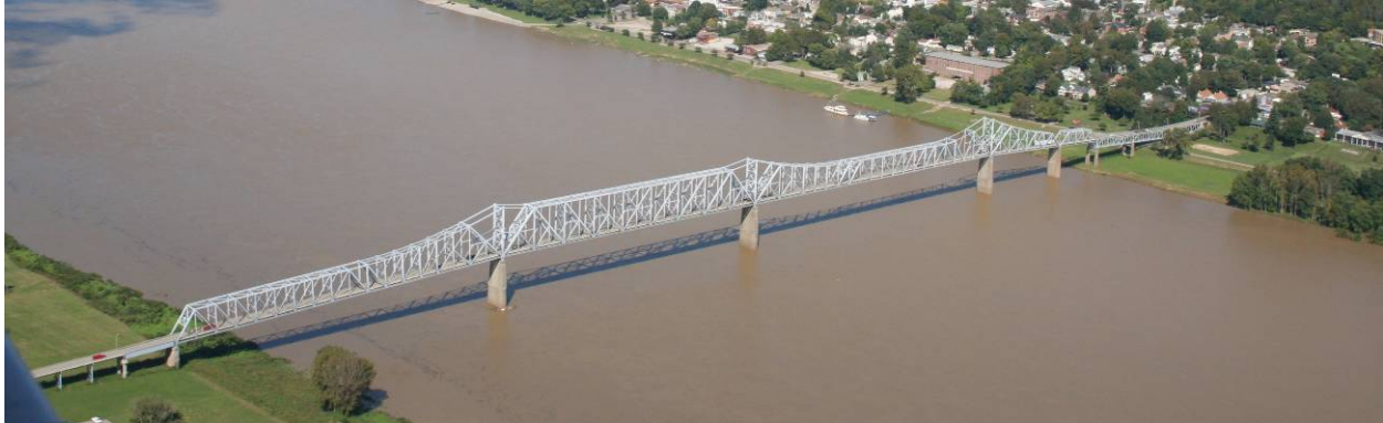
The existing US 421 Milton-Madison Bridge
