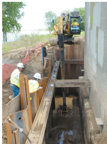
Pier strengthening is underway.
