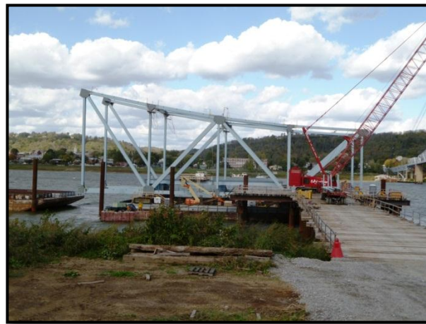
A 600-foot span is being preassembled on barges.
